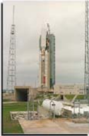
Titan launch vehicle on the pad at KSC (Photo: USAF)
